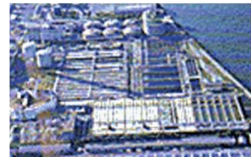
Hiagari Purification Center Start of Operation: April 1970
