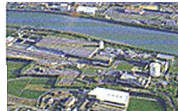
Sone Purification Center Start of Operation: October 1979
