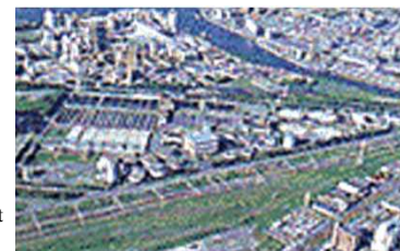
Kogozaki Purification Center Start of Operation: July 1963
