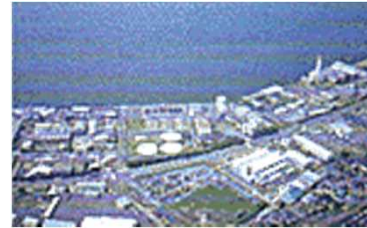
Shinmachi Purification Center Start of Operation: April 1972
