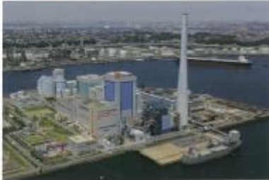
Large scale power plant boiler Photo courtesy of JPO/ST/1503
