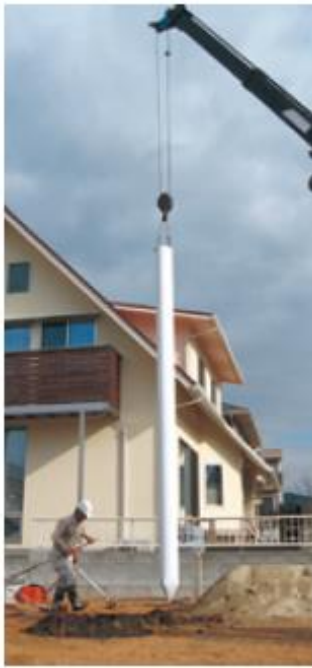
Installing a Geo Pipe in the ground. Pipe length: 5 to 7 meters.
