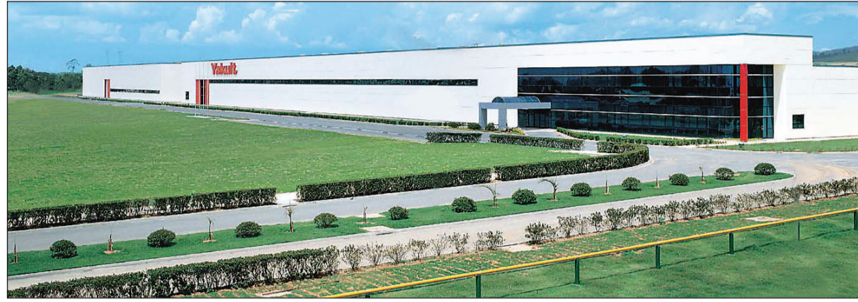
Yakult's third centralized production facility at Lorena, Sao Paulo
